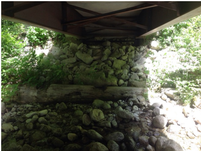
Right Bank Abutment when facing downstream
