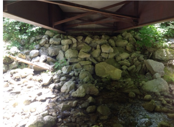
Left Bank Abutment when facing downstream
