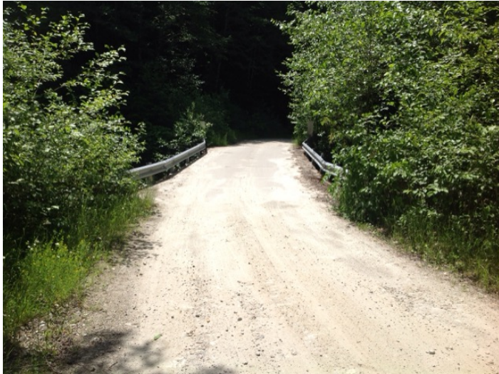
Approach from Right Bank when facing downstream
