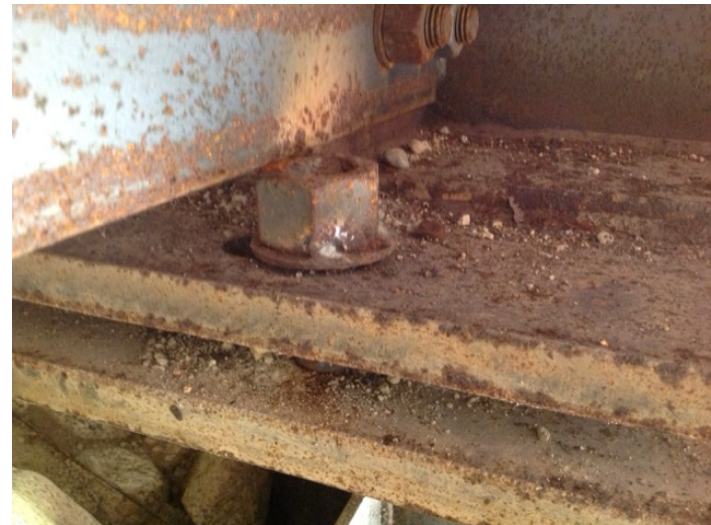
bearing plates at extent of slot
