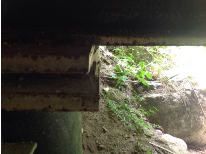
bearing plates offset 14mm
